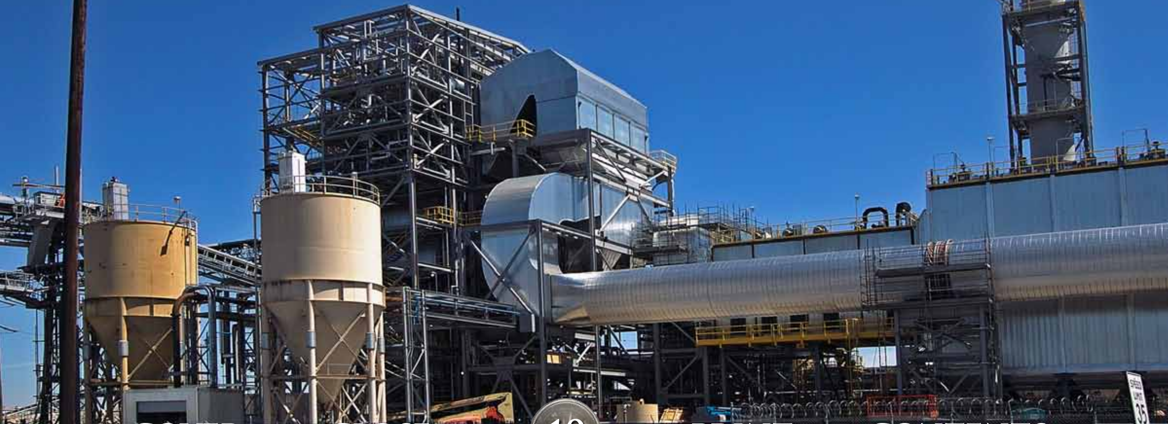
DTE Energy under construction.
